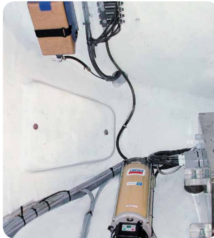
Lubrication System including pump 603S, QSL and SE1 suction element and used lubricant container
